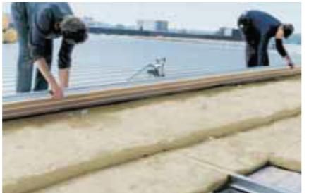
Special aluminium clips have to be used for joining the Kalzip® profiled sheets with the substructure of the roof. They are locked into the seam and will be overlapped by the following Kalzip® element, so that the fixing elements are hidden under the roofing. This ensures that the roofing elements need not to be punctured for fastening.
